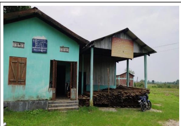
Common facility center: Kakopathar, Assam
