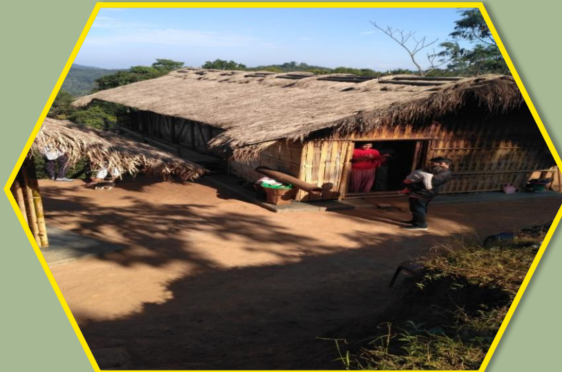
Cane and bamboo construction
