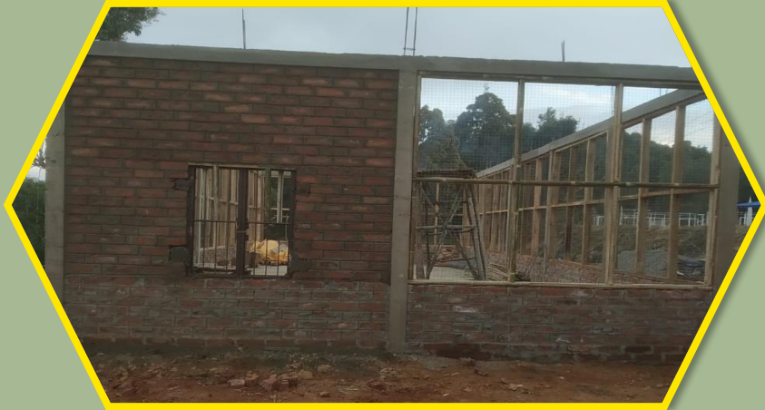
Construction of Common Facility Centre
